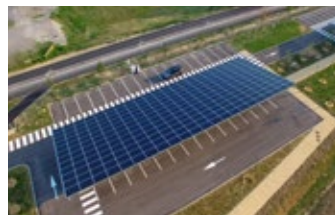
Ombrières photovoltaïques du parking inter-entreprises
